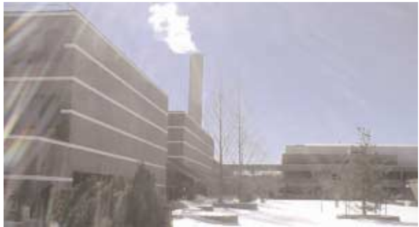
Rockland Community College's Main Utility Plant
