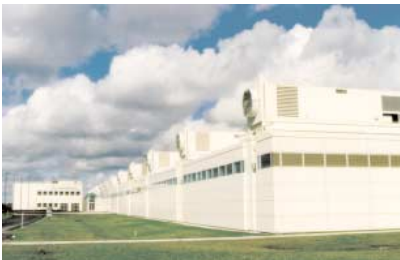
Roof-top air-conditioning units at the Elma facility.
