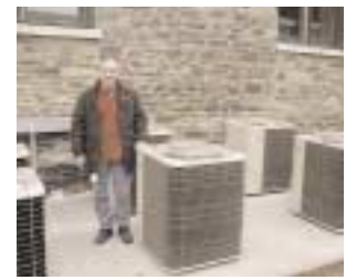
Equinox project architect Frances Kramer stands beside multiple HVAC units.
